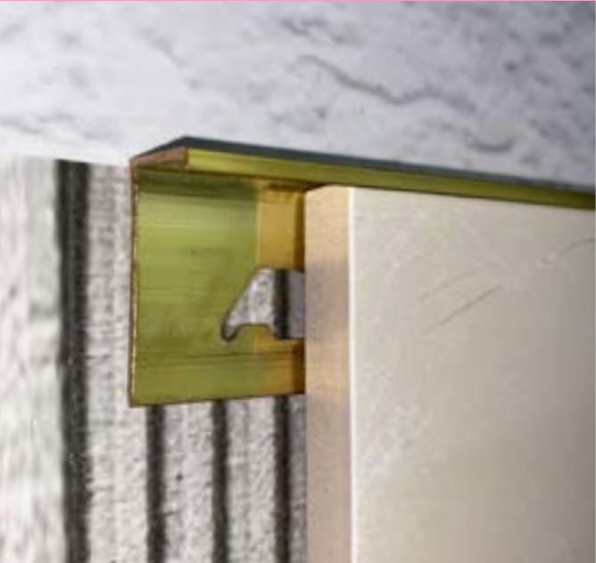
Chiusura perimetrale a muro/ Wall covering edging
